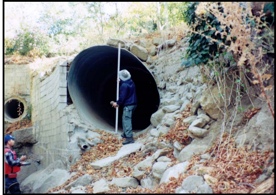
Right Culvert Outlet
