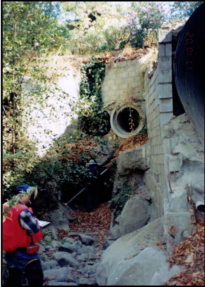
Left Three Culvert Outlets
